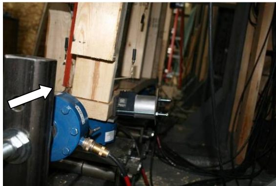
Photo 1: Stud/Plate Separation at Hold Down
