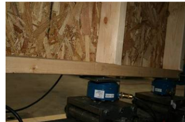
Photo 32: Base Bearing Plate
