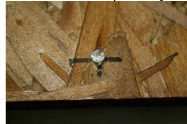
Photo 23: Sheathing Fastener Placement
