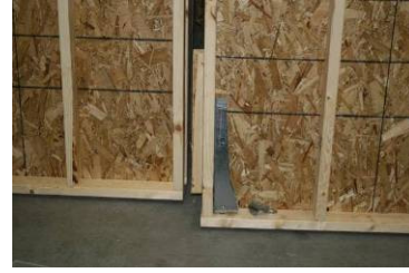
Photo 27: Simpson HDU8 Hold Down
