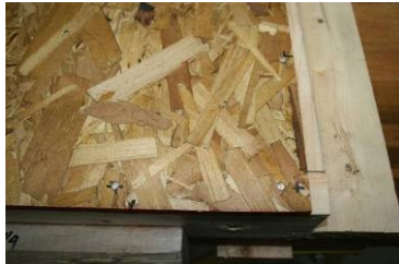
Photo 22: Sheathing Fastener Placement
