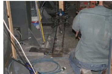
Photo 34: Alignment of Frame
