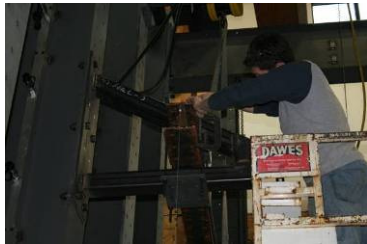
Photo 33: Alignment of Frame
